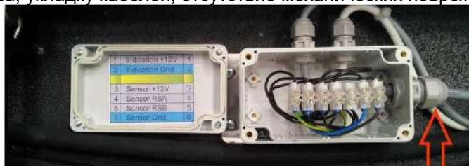
Checking the leaktightness of the connection boxes and sealed cable inputs
